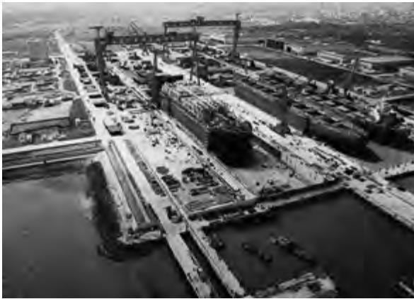
Figure 1. A 2G shipyard characterised by its goliath cranes and graving docks. These assets and the piers and wharves are permanent fixed and will have to be demolished when the industry fails. (Image: Courtesy of Waigaoqiao Shipbuilding China)
