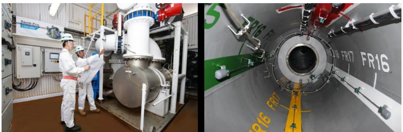
Figure 6: Sembcorp Marine environmental products: Semb-Eco LUV ballast water management system (left); Semb-Eco ElMag Corrosion Protection System applied to VLCC stern tube (right).
