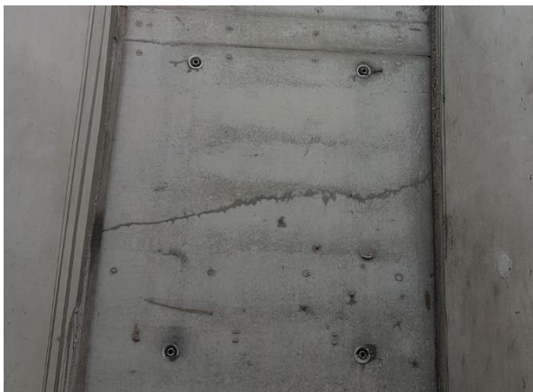
Figure 2: Restraint cracking on fresh concrete cast in-between two precast members
